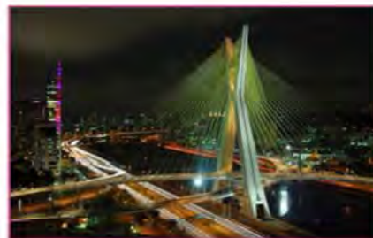
Ponte Estádio Octávio Frias de Oliveira http://www.skyscrapercity.com/member.php?u=449572
